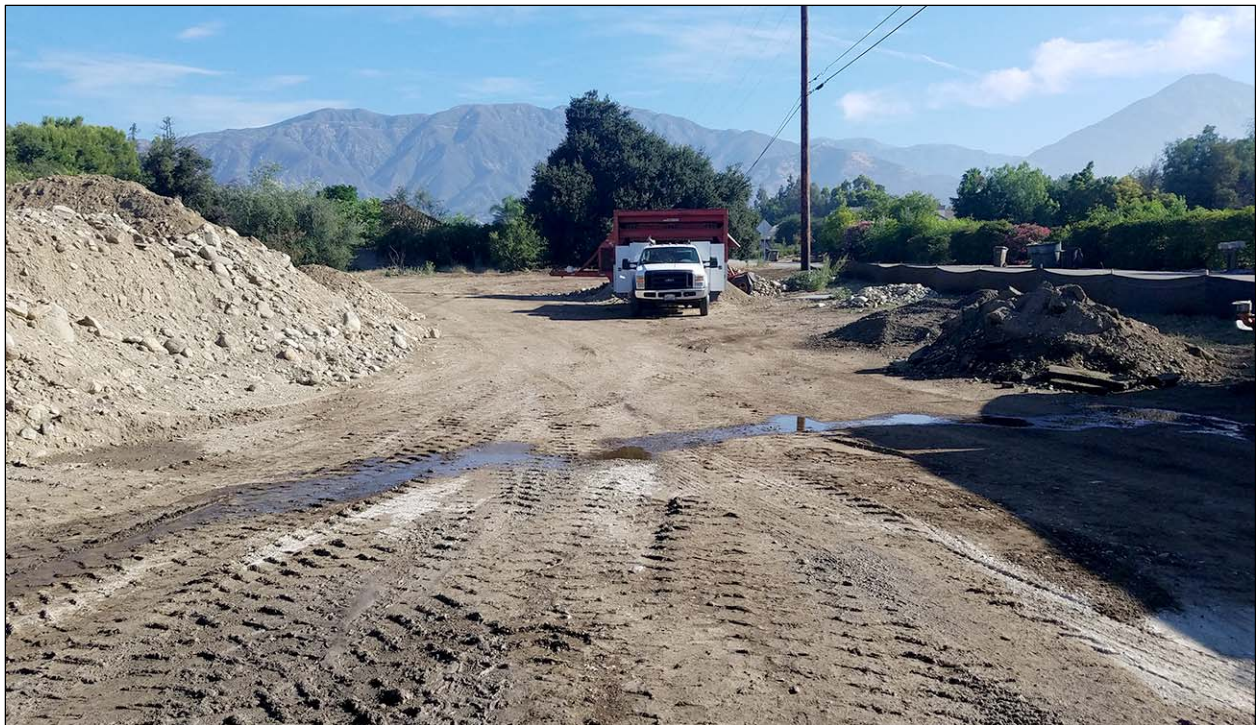
Figure 4. Overview of the project area. (Photograph taken on July 29, 2019; view to the north)
